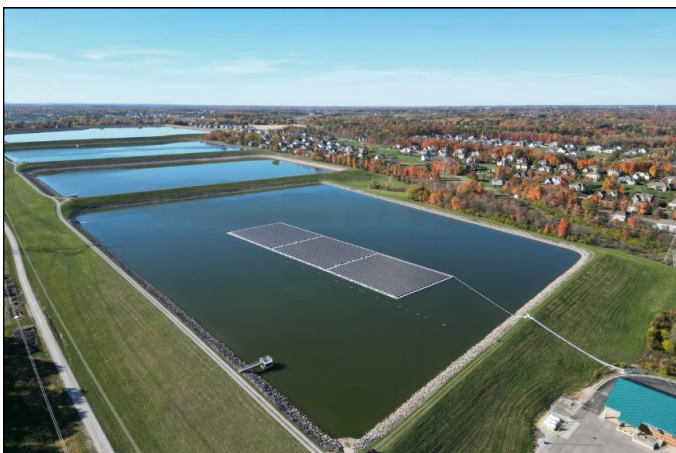
Del-Co Water Headquarters on S.R. 315, Liberty Township—Reservoirs
