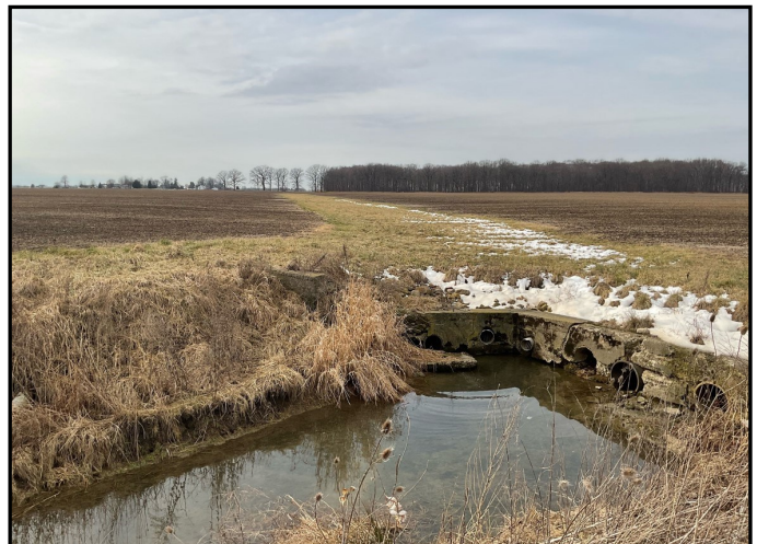
Source: DSWCD Project: Thomas Agricultural Drainage
