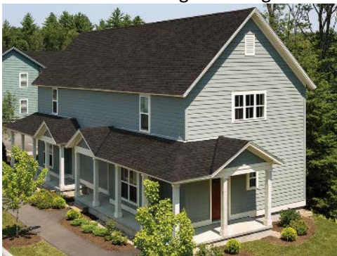
Gable Roof: From iko.com
