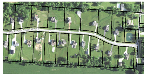
Estates at Cheshire is a traditional subdivision utilizing FR-1 zoning on S. Galena Road.
