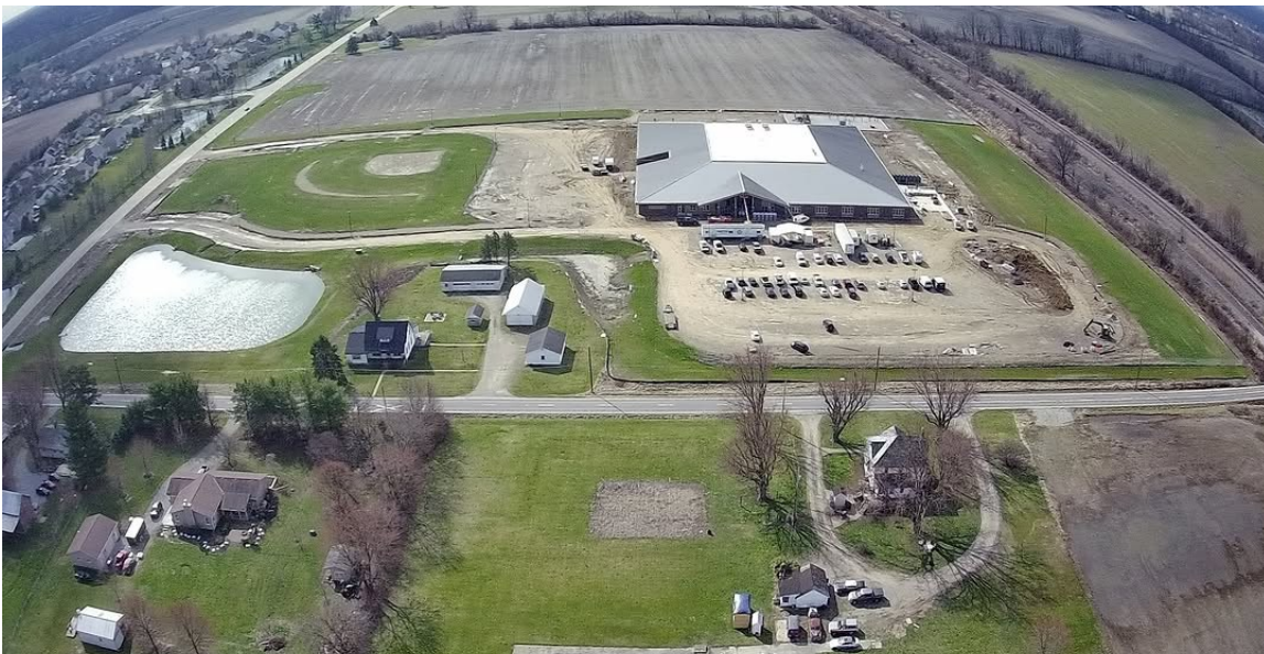
Peachblow Crossing Elementary School during construction, Berlin Township
