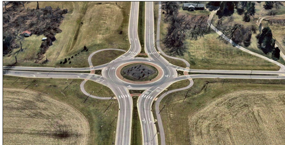
The roundabout at Bunty Station provides an opportunity for township identity through signage and enhanced landscaping.
