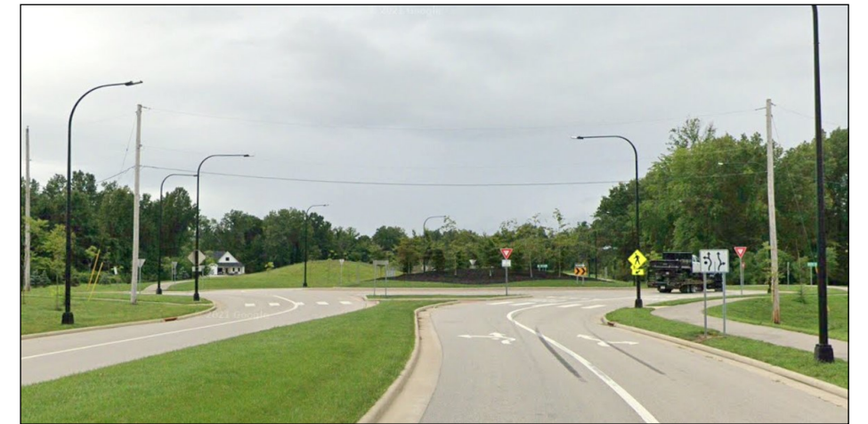
Bunty Station roundabout from the north.
