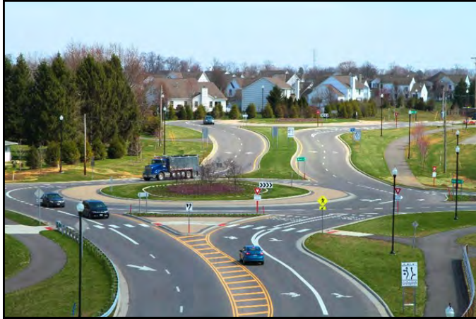
Modern, low-speed roundabout; South Section Line Road and Riverside Drive, Concord Township. Pedestrian crosswalks are behind the pause line for traffic. Safe design speed is 11 miles per hour.
