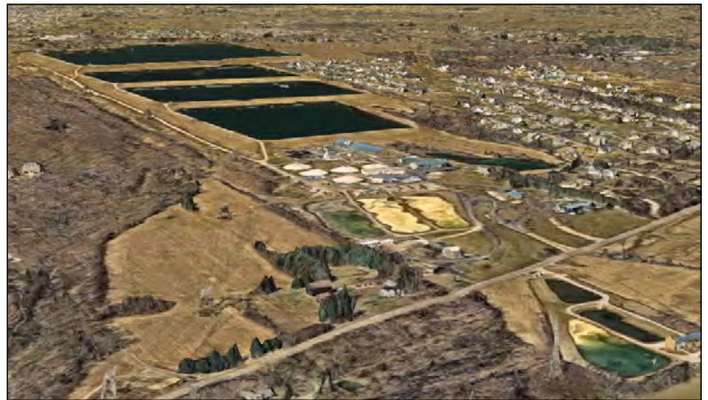
Del-Co Water Headquarters on S.R. 315, Liberty Township
