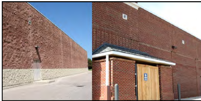
Blank walls (left) should include architectural detail (right), although windows and doors are preferred.
