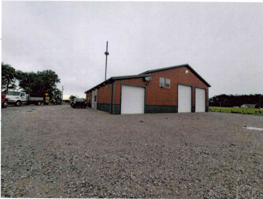
Photograph of the south side (back) of the existing building.
