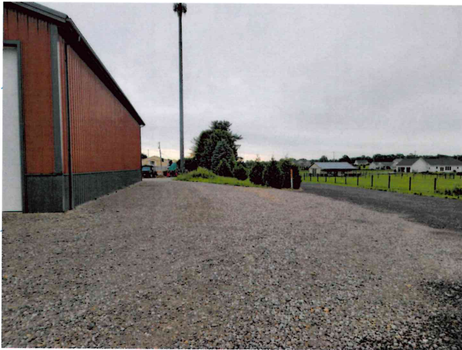
Photograph looking north along the east edge of the building showing nearest residence.
