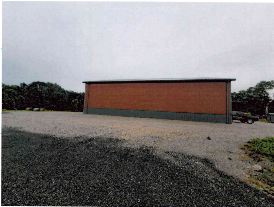
Photograph of east side of the building, toward residential lots.
