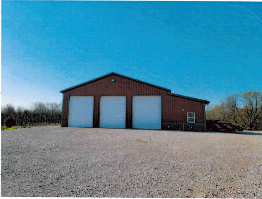
Photograph of the north side (front) of the existing building.
