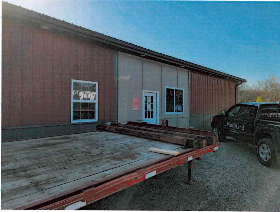
Photograph of the west side (office entrance) of the existing building.
