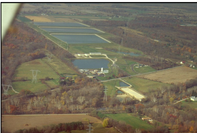
Del-Co Water Headquarters on S.R. 315, Liberty Township
