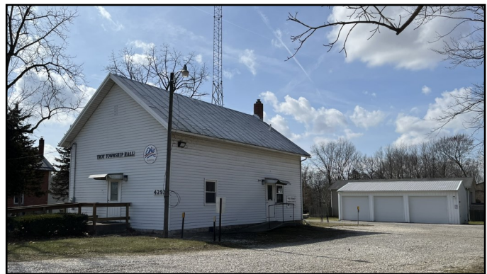
Figure 10.13. Troy Township Hall and Maintenance Building
