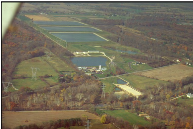
Del-Co Water Headquarters on S.R. 315, Liberty Township
