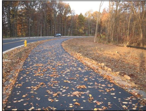
Multi-use path near the Tanger Outlets
