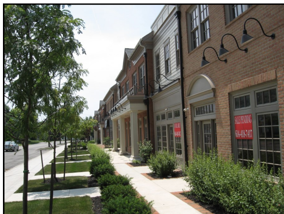
“In-line” stores, or strip centers, built with high-quality materials and architectural details
