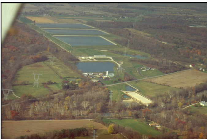
Del-Co Water Headquarters on S.R. 315, Liberty Township
