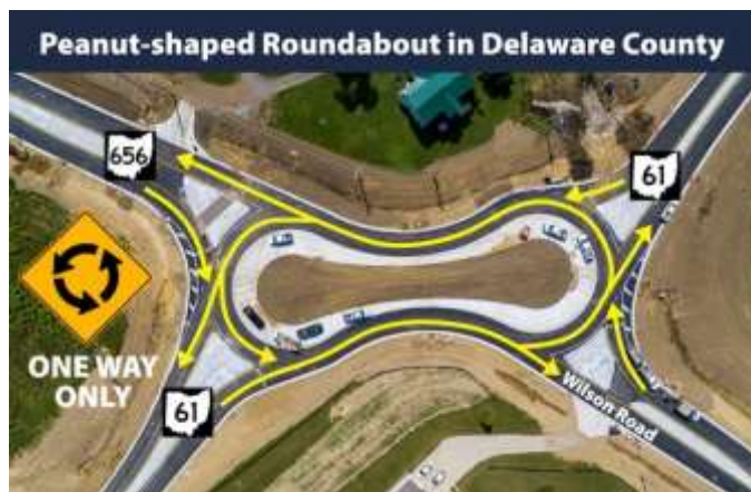
ODOT completed construction of a peanut-shaped roundabout at the intersection of State Route 61 and SR 656/Wilson Road. In addition to reducing crashes by 70 percent, the safety upgrade is expected to improve traffic flow at the intersection. The $2 million safety project began in May 2021 and opened to traffic Monday, August 9, 2021.
