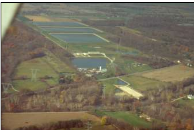
Del-Co Water Headquarters on S.R. 315, Liberty Township
