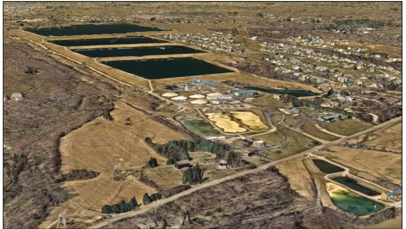
Del-Co Water Headquarters on S.R. 315, Liberty Township
