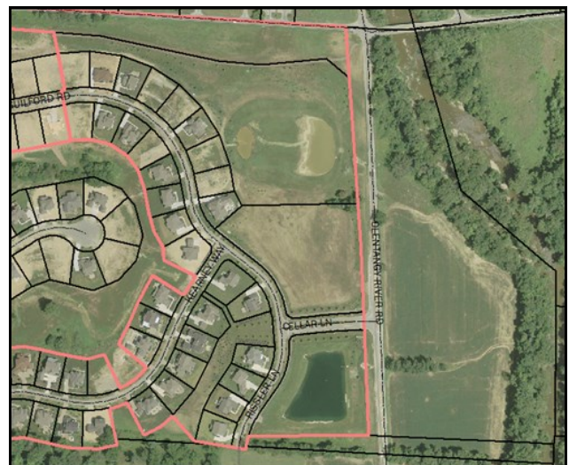
A portion of Trail’s End subdivision Although developed under the PR standards, the project includes many features of a Conservation Subdivision (see next section).
