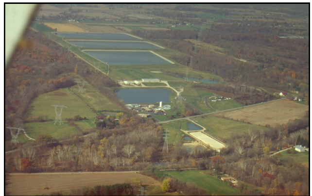
Del-Co Headquarters, S.R. 315
