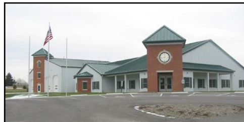
Scioto Township Hall and Fire Station.
