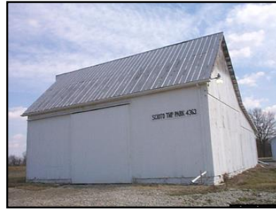
Structures within the 35-acre Scioto Township Park.
