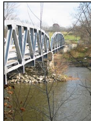
Warrensburg Road bridge over the Scioto.
