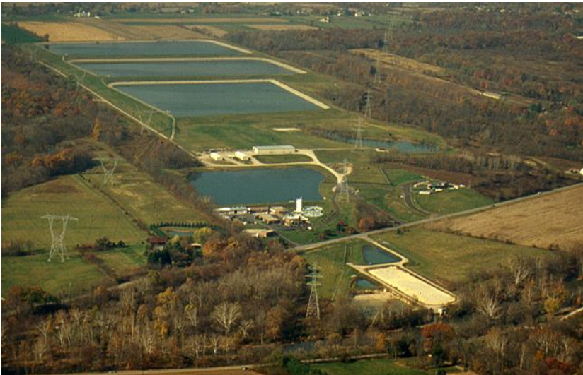
Del-Co Water Headquarters and Up-Ground Reservoirs on State Route 315, Liberty Township.
