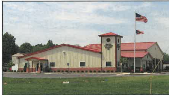
The Fire Station – corner of Lackey Old State and Cheshire Roads.
