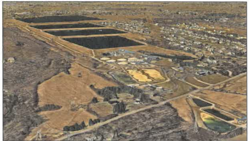
Del-Co Water Headquarters on S.R. 315, Liberty Township
