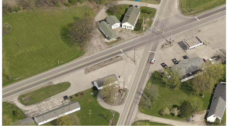
Intersection of South Section Line and U.S. 42.
