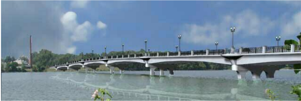
The Home Road Bridge at Rathbone
