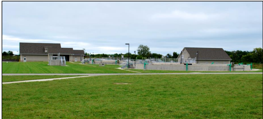
Lower Scioto Wastewater Treatment Plant.
