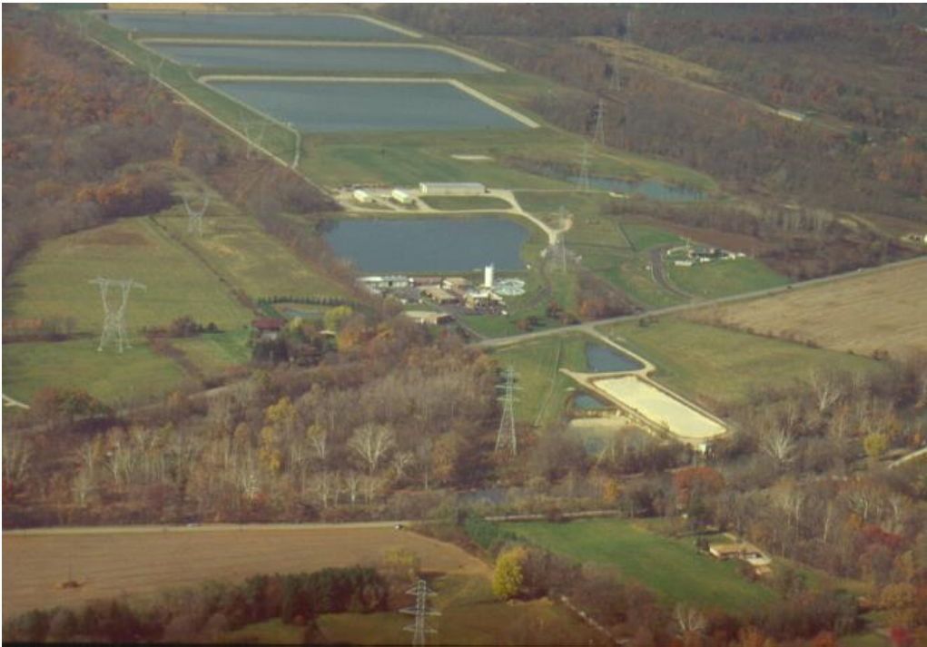
Del-Co Water Headquarters and Up-Ground Reservoirs on State Route 315, Liberty Township
