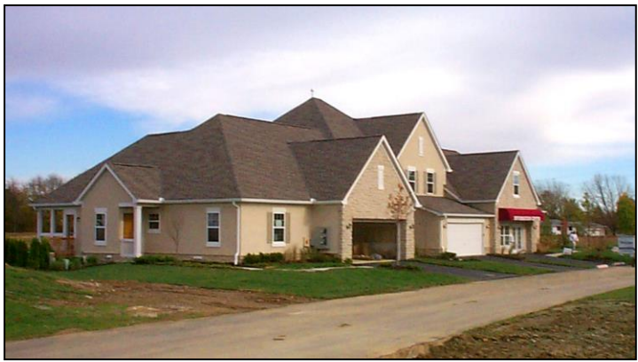
Multi-unit condominium development.
