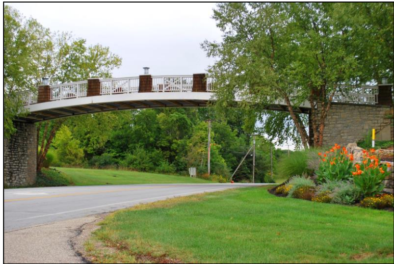
Bridge over Concord Road at Tartan Fields.
