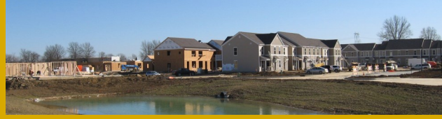
Orange Grand is a multi-family project that started construction in 2019.
