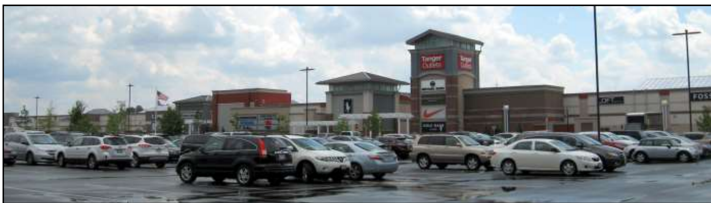
Simon Tanger Mall in Berkshire Township
