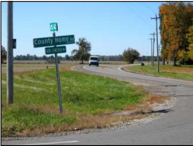
Rural roads are predominant in Brown Township.
