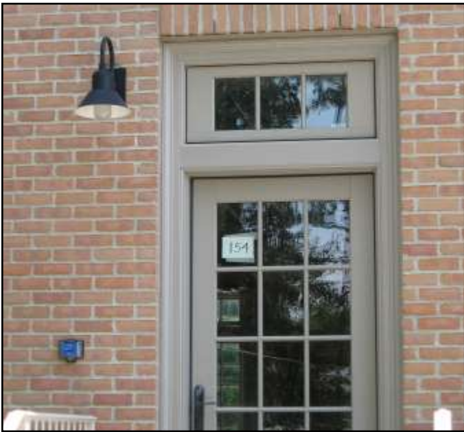
Example of lighting designed as a cohesive part of other site elements
