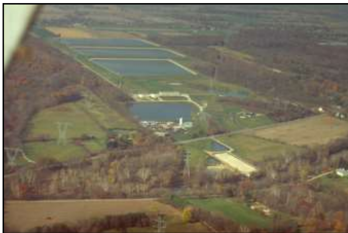
Del-Co Water Headquarters on S.R. 315, Liberty Township
