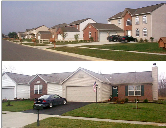
Examples of snout houses; two story houses on 75' frontage (top) and single-story houses on 50' frontage.
