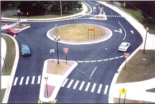
Modern, low-speed roundabout. Pedestrian crosswalks are behind the pause line for traffic. Safe design speed is 11 miles per hour. Location: Michigan, design by DLZ Engineers.
