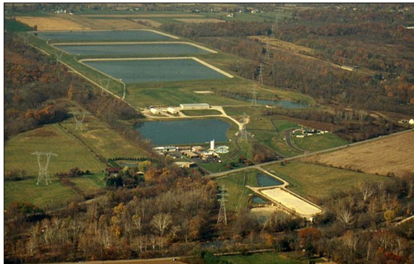
Del-Co Water Headquarters and Up-Ground Reservoirs on State Route 315, Liberty Township. A 1 billion gallon reservoir has been added since this photograph was taken.
