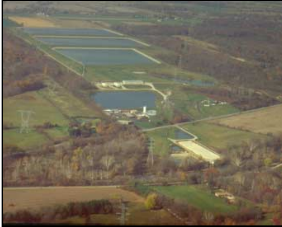
Del-Co Water Headwaters and Up-Ground Reservoirs on State Route 315, Liberty Twp.
