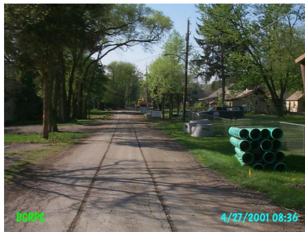
Pavement scored in preparation for sewer trenching, 2001
