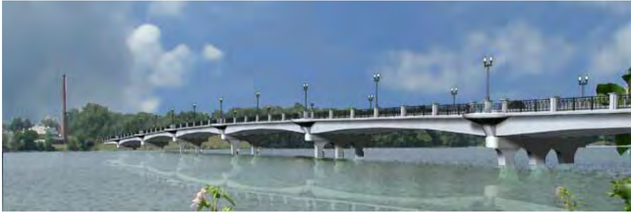
The Home Road Bridge at Rathbone
