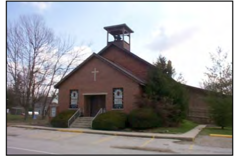
Church in Bellepoint.
