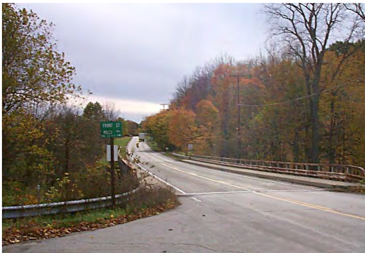
Mills Road and S.R. 257 in Bellepoint
