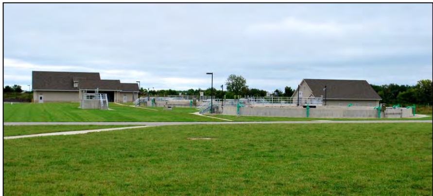
Lower Scioto Wastewater Treatment Plant.
