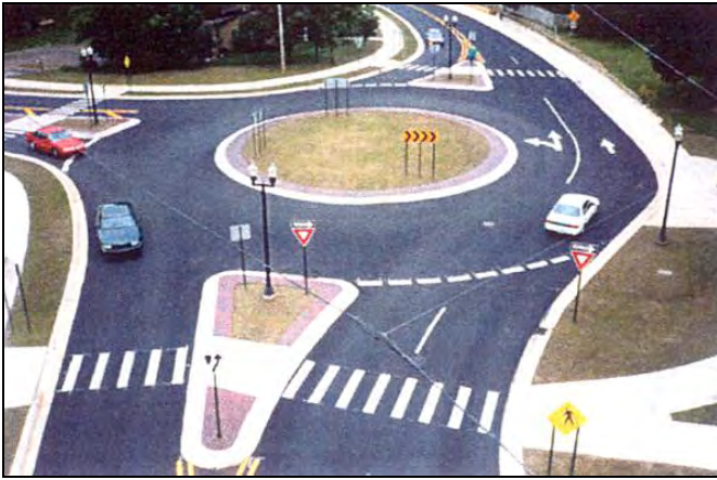
Modern, low-speed roundabout (DLZ Engineers)
