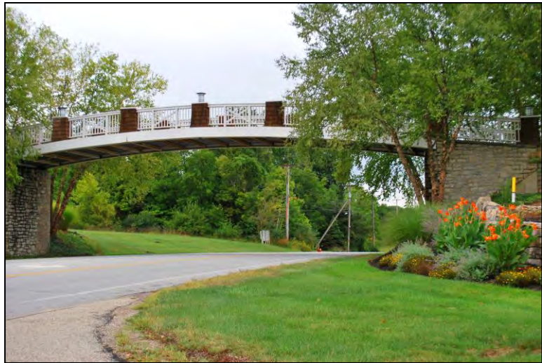
Bridge over Concord Road at Tartan Fields.
