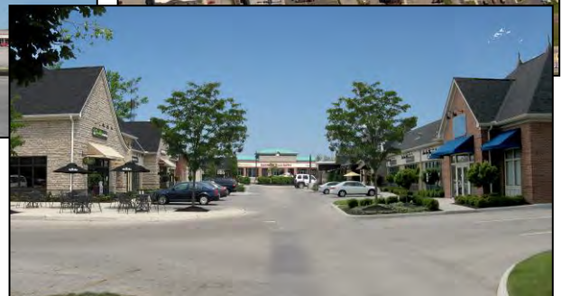
The under-utilized parking area between Wal-Mart and Kohl's on U.S. 23 (top) is filled with a set of in-line stores (middle). The featureless lot (left) becomes a pedestrian-oriented feature of the site (above).
