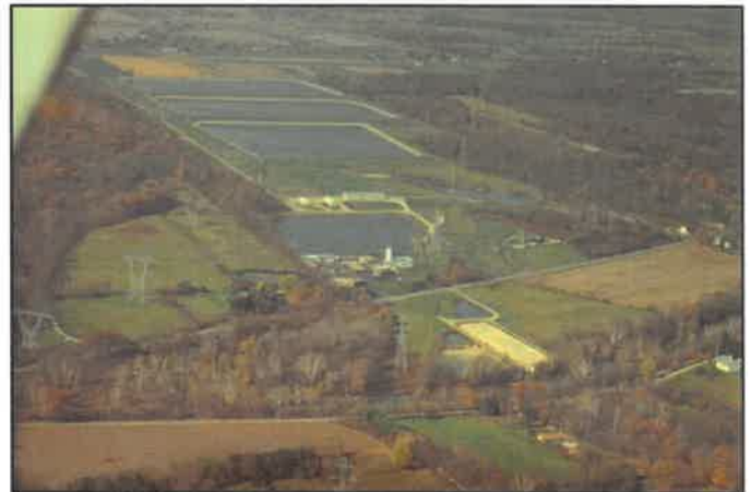
Del-Co Water Headquarters on S.R. 315, Liberty Township
