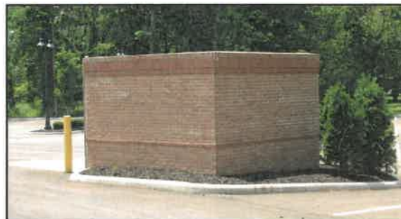
Example of screened dumpster
