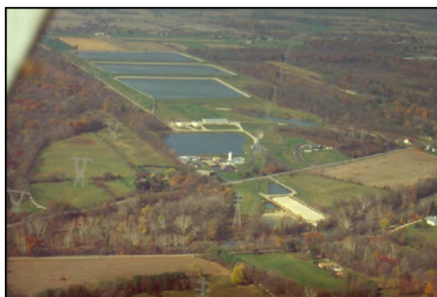
Del-Co Water Headquarters on S.R. 315, Liberty Township
