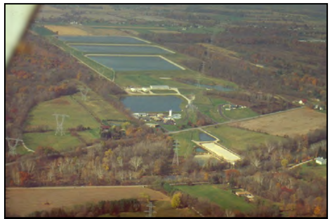
Del-Co Water Headquarters on S.R. 315, Liberty Township
