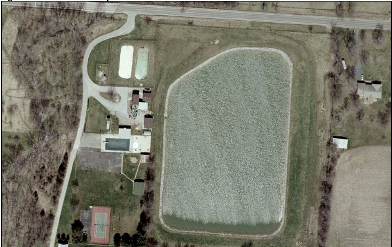
Figure 10c. Aerial of Ashley's Water Treatment Plant
