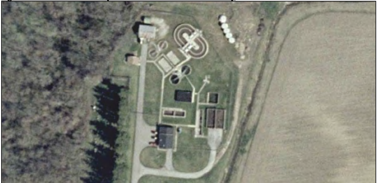
Figure 10a – Aerial of Ashley's Wastewater Treatment Facility
