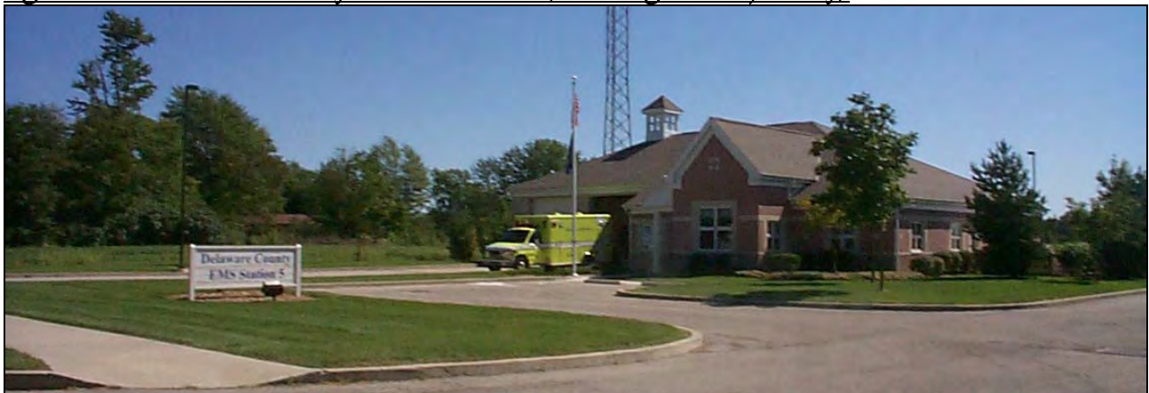
Figure 11d. Delaware County EMS Station #5 (West High Street, Ashley)
