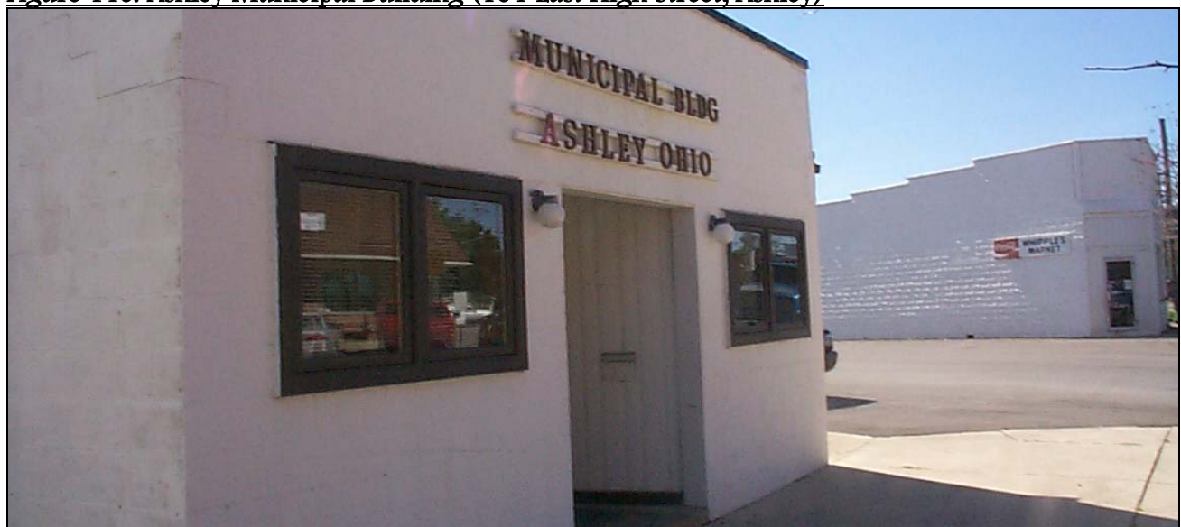
Figure 11e. Ashley Municipal Building (101 East High Street, Ashley)
