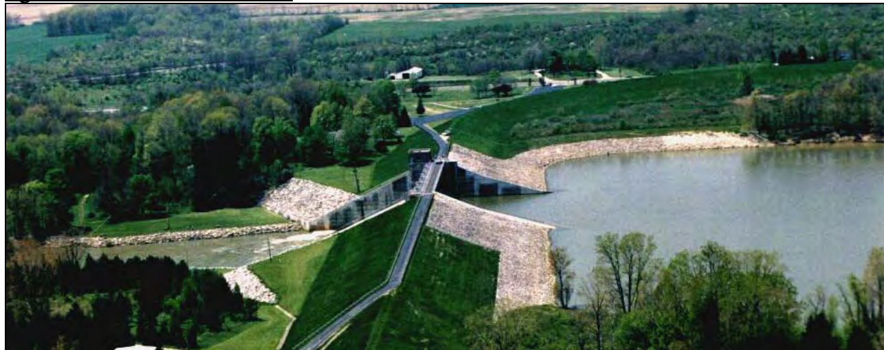
Figure 12f. Delaware Dam Area
