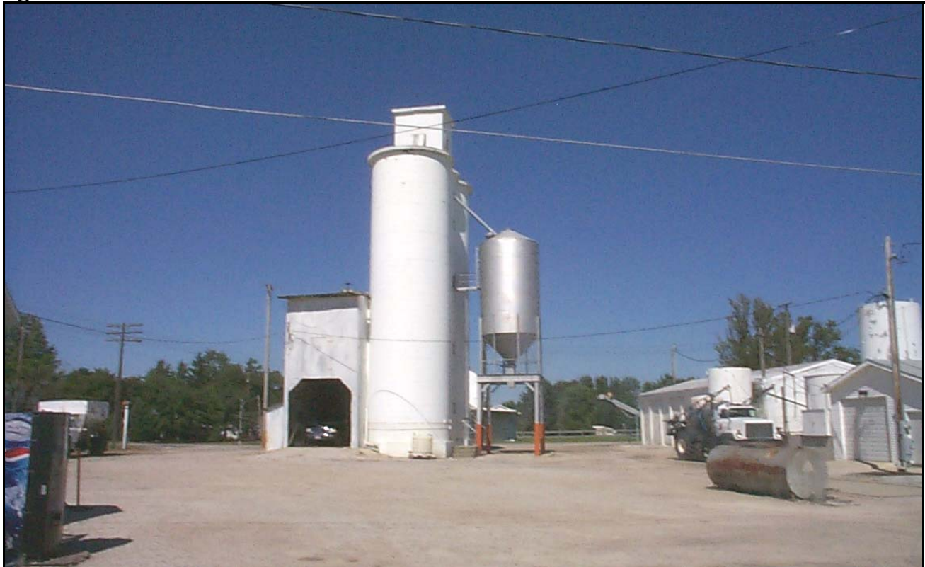
Figure 8a – Marion Landmark Grain Elevator
